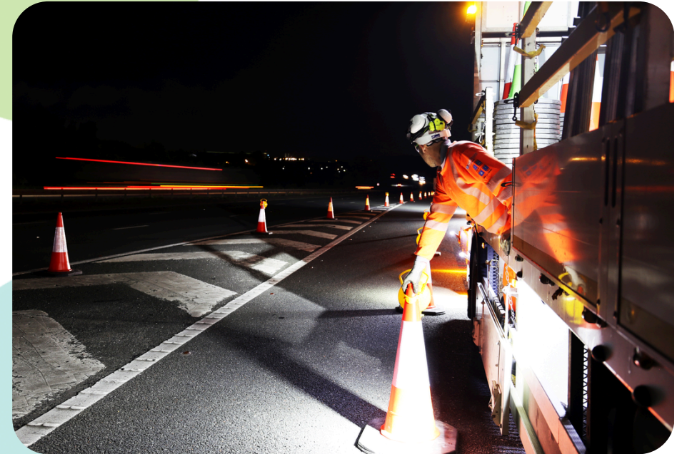
Contractor for KCC Highways
